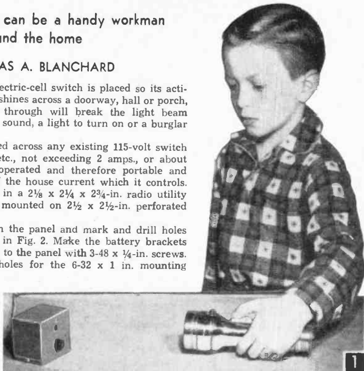
Tiny self-contained photoelectronic control being test-actuated at close range with flashlight. Unit is sensitive enough to respond to feeble daylight at surprisingly long distances.
